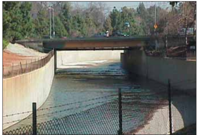
Figure 2.1 Existing condition at Studio City (Photo by Nuvis Landscape Architects)
