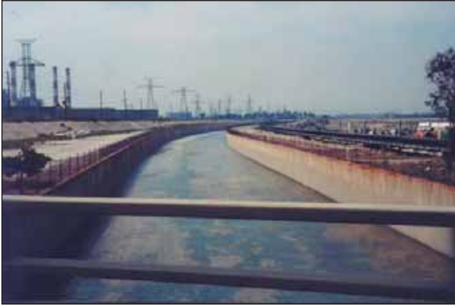
Figure 2.5 Existing conditions on Tujunga Wash
