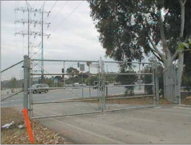
Figure 14.9 Maintenance gate alternative by City of Los Angeles Department of Transportation. Five bar vehicular maintenance gate at Los Feliz Bike Path.
