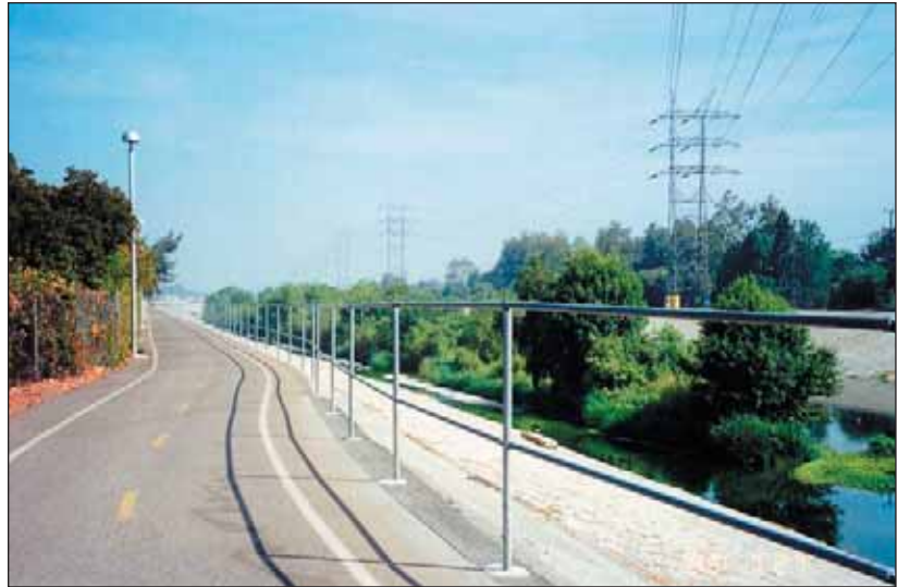
Figure 14.48 Class I Bike Path with fence at Glendale Narrows.
