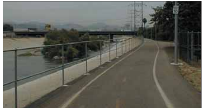
Figure 5.5 City of Los Angeles Bike Path, west bank, fencing on trapezoidal channel
