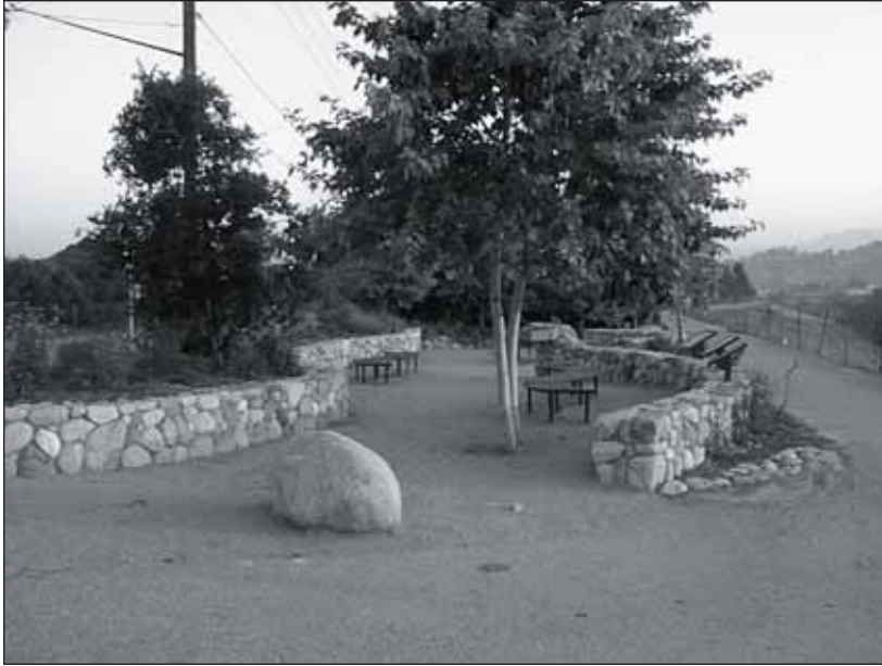
Figure 14.36 Freestanding stone seatwall at Egret Park at Riverside Drive, City of Los Angeles.
