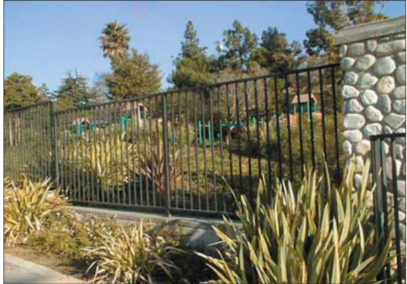
Figure 14.2 Tubular steel fence application with arroyo stone accents. Installation to be done in accordance with manufacturers specifications.
