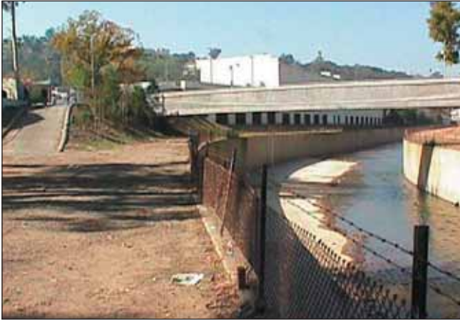
Figure 2.3 Existing conditions between Whitsett Avenue and Laurel Canyon Blvd. (Photo by Nuvis Landscape Architects)
