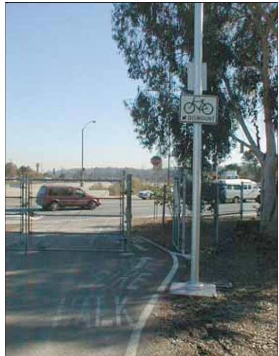
Figure 14.56 Bicycle dismount sign mounted on light pole at Los Feliz Boulevard.
