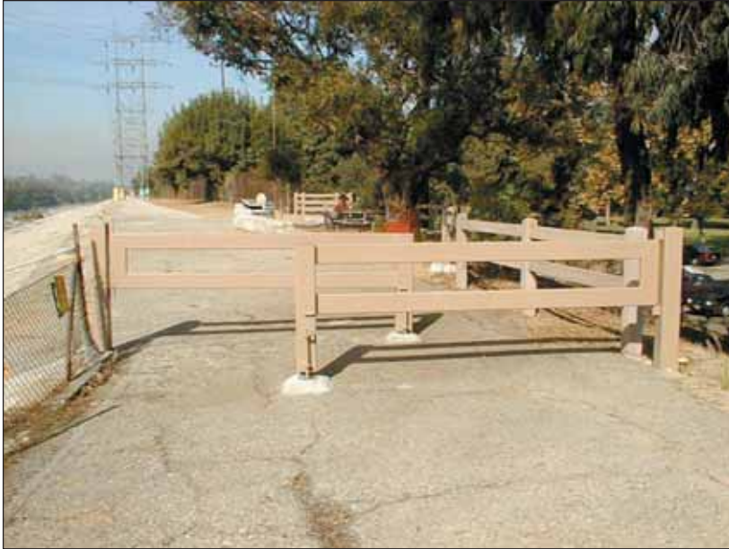
Figure 14.17 Custom steel swing gate designed and installed by North East Trees at Los Feliz Boulevard for equestrians.
